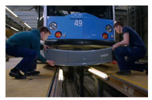
Installation of the 3D printed housing cover
